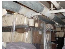
File storage in the basement of the Multnomah County Courthouse.
